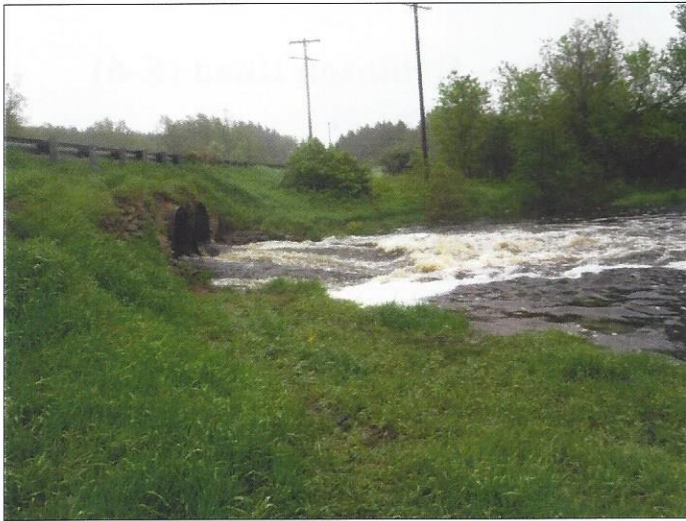
Before - The inadequate twin culverts impeded fish passage and roadbed runoff contributed excessive sediment to the stream
